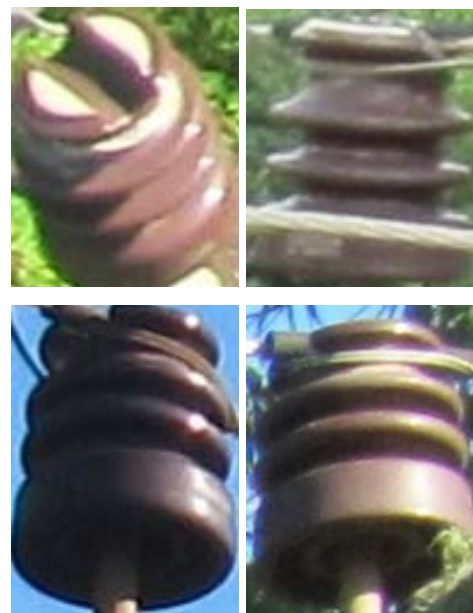
Fig. 1. Insulators considered suitable for working.
