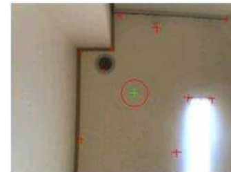
(a) Molding edge between ceiling and wall
